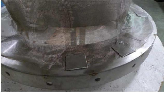
The stainless steel net should be extended around the gap where the expansion joint will be placed (around the metal shirt in case it exists).
