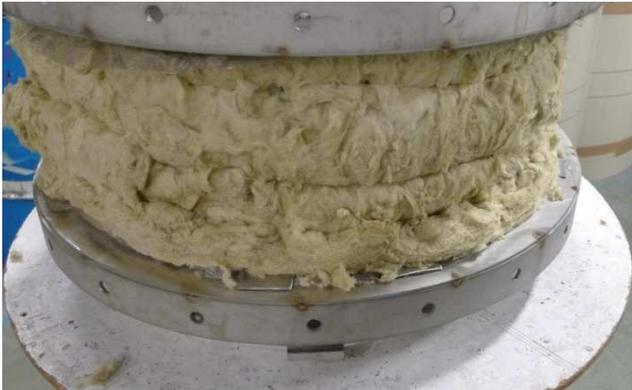
The first layer of rock lane should be placed around all the diameter of the assembly.
